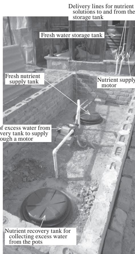
**Fig. 6** Underground supply of fresh water nutrients and recovery tanks of 1000 liter capacity in closed loop along with transfer motor.
