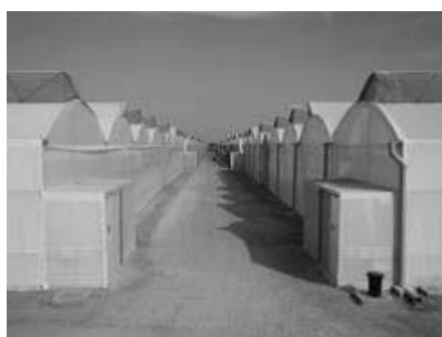
Fig. 13 Computer-controlled greenhouses with (Left) ridge vents for ventilation and (Right) fogging nozzles for cooling and thermal screens to reduce sun light (currently, they are wide-open)
