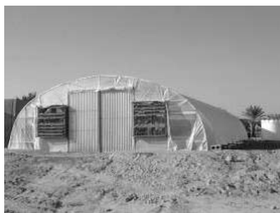
Fig. 10 Fan-pad evaporatively cooled greenhouse (Al-Ismaili, 2003)
