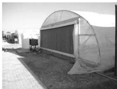
Fig. 10 Fan-pad evaporatively cooled greenhouse (Al-Ismaili, 2003)
