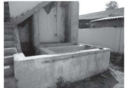
**Fig. 17** Cement concrete tanks constructed along the wall of an existing building for three stage washing of ginger.
