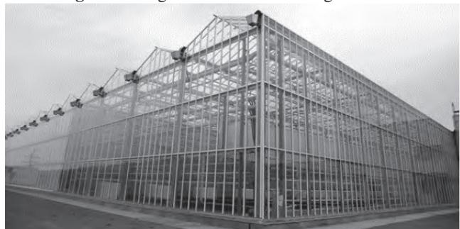
tage of this type of greenhouse is that it is unable to sustain an optimum microclimate during the warm period of the year. Because there is no system to reduce the internal temperature, the risk of over-heating is high (Fig. 3)
